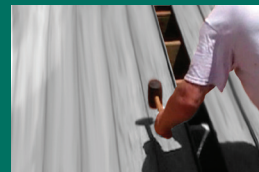
Lay Down Deck Board
